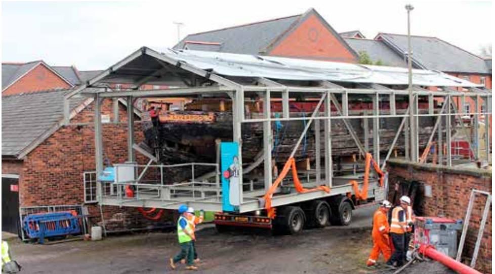
Mossdale loaded on the lorry, ready to be manoeuvred into position
