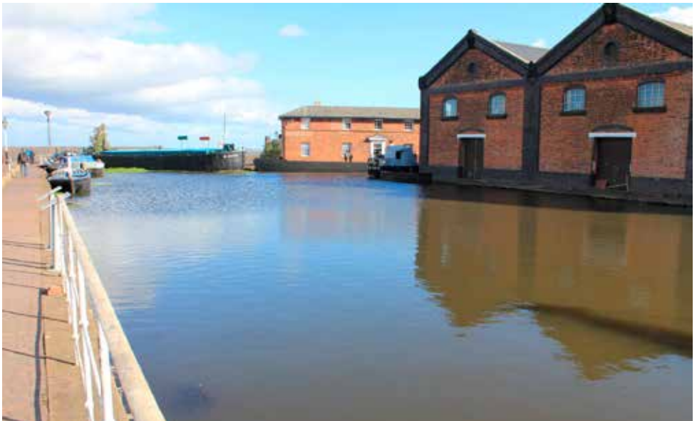
... and after the job was complete
