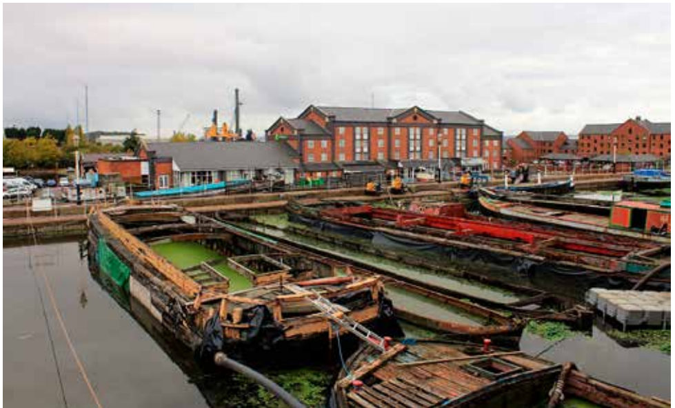
The Top Basin prior to the boats being lifted...
