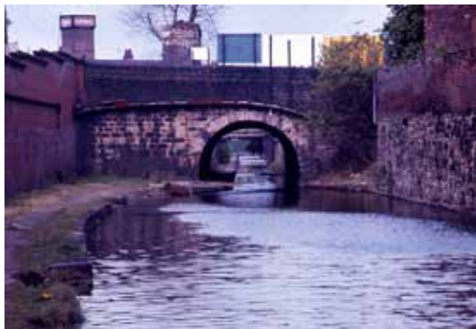
Looking back, whilst the canal was still un navigable in 1974, towards the first lock, through the former Whitelands Tunnel photo: Chris Griffiths
