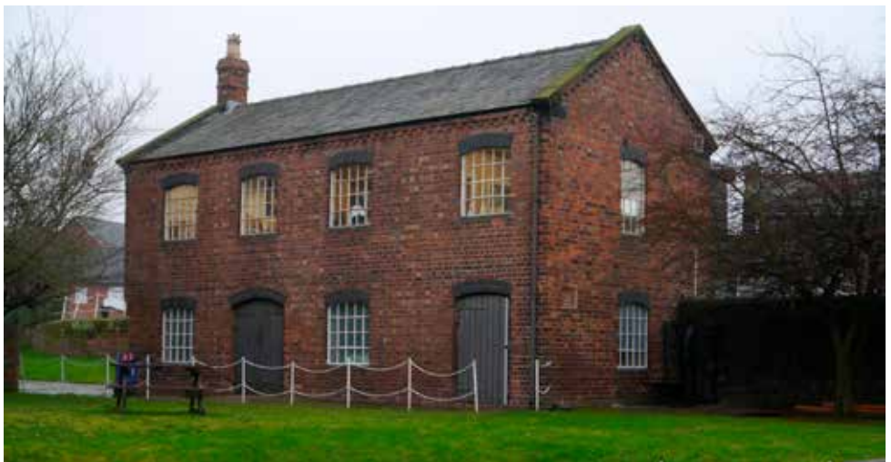
The two-storey rear elevation of the building
